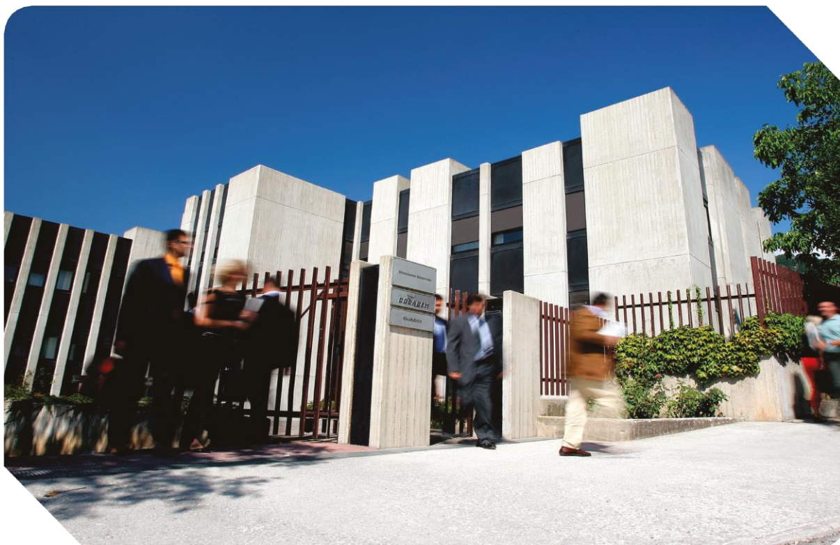
Figure 1 – Headquarters of Colacem S.p.A. - Gubbio (PG)
